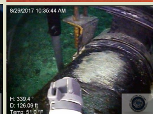
Above: Diagram of anchor support installation. Lower right: Bare metal of pipe adjacent to anchor support. Lower left: Calcareous deposit on pipe line.
