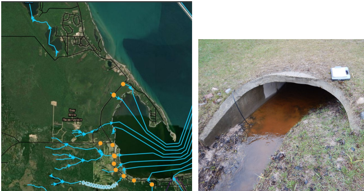
Figure 6a. Road-stream-crossing locations around Waishkey Bay. Many more driveway and ditch culverts exist, but were not assessed. Figure 6b. High priority crossing 281/282 at BMRC.
